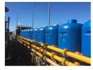
The ZTPS™ is a treatment plant that recovers 99-99.5% of the methane from the raw BioGas.
